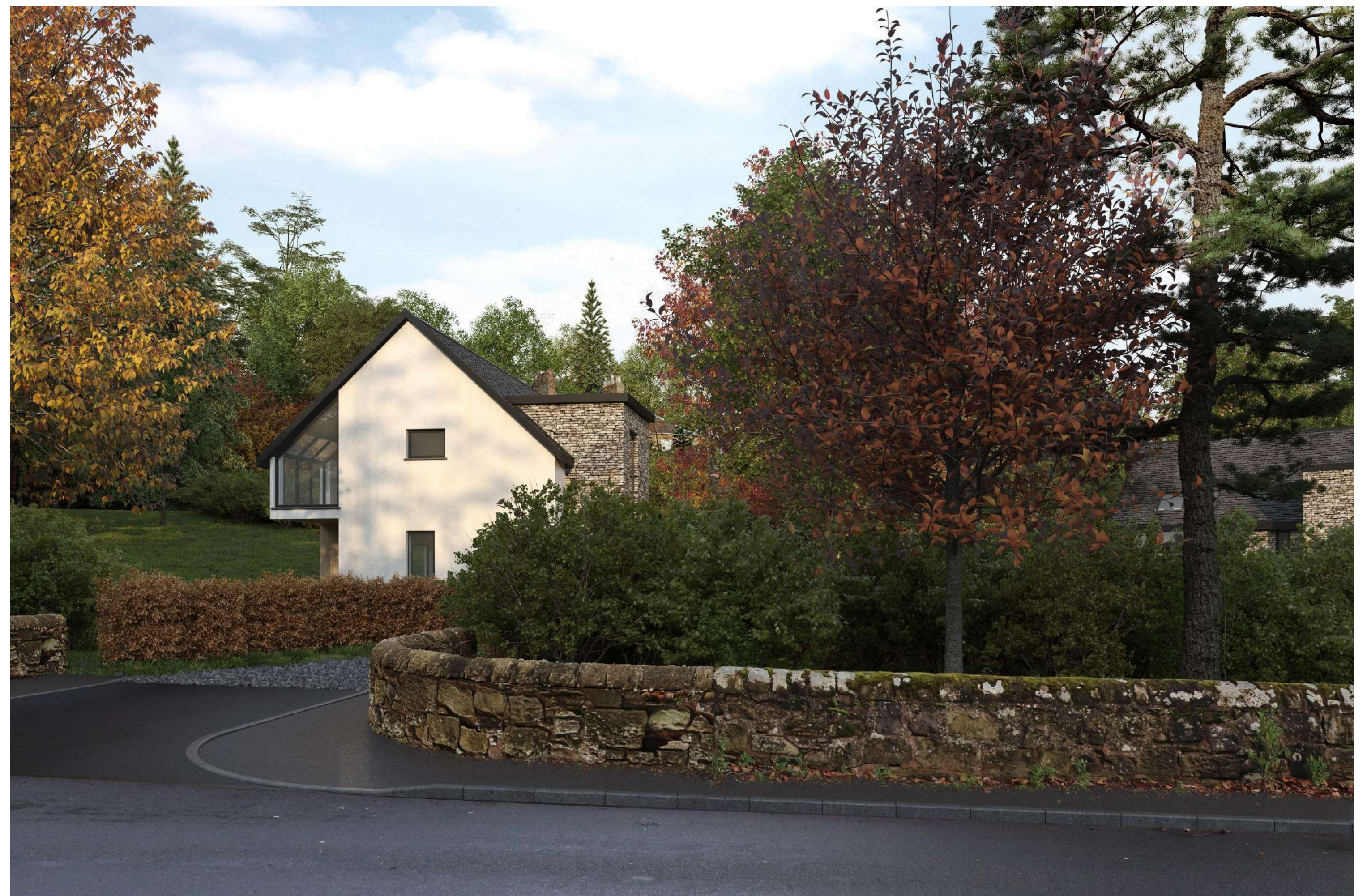
VIEW POINT B2 – 5 YEARS POST COMPLETION
